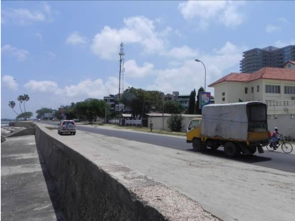
Figure 6: Relation of the current sea wall to Ocean road and other infrastructure
