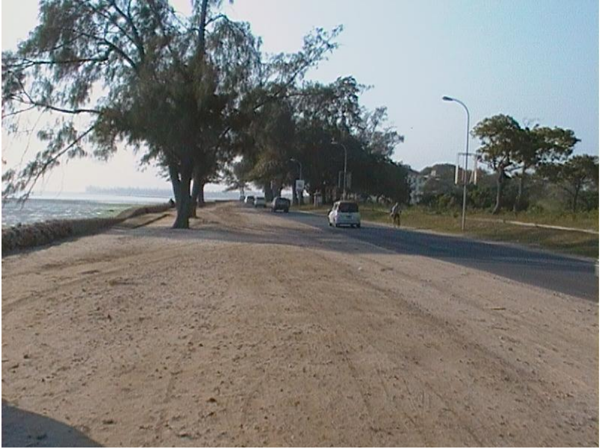
Figure 8: Ocean Road. Some stretches directly behind the sea wall are left bare, or with only sparse vegetation.
